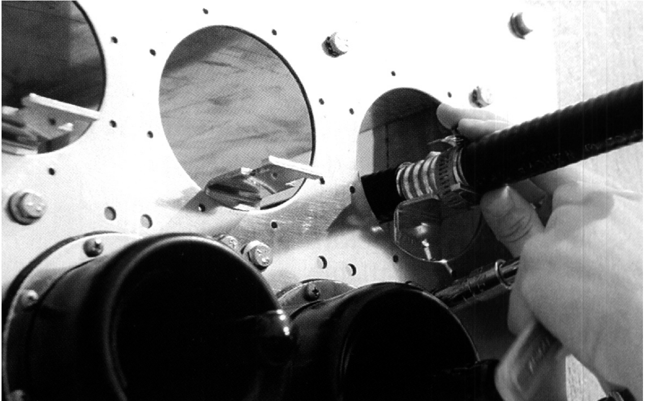
Figure B7 - Exterior View Of Coax Cable Multiport Entry Bulkhead
