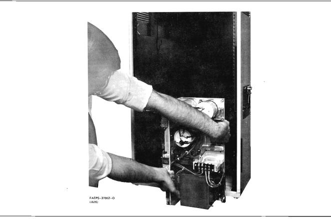
Figure 5. Power Supply Removed From Cabinet
