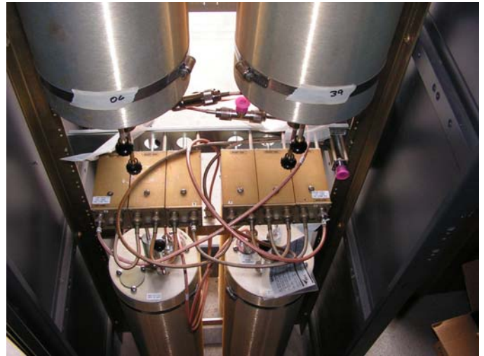
Figure 2 — The second duplexer used as the combiner to add digipeater capability to the system.
